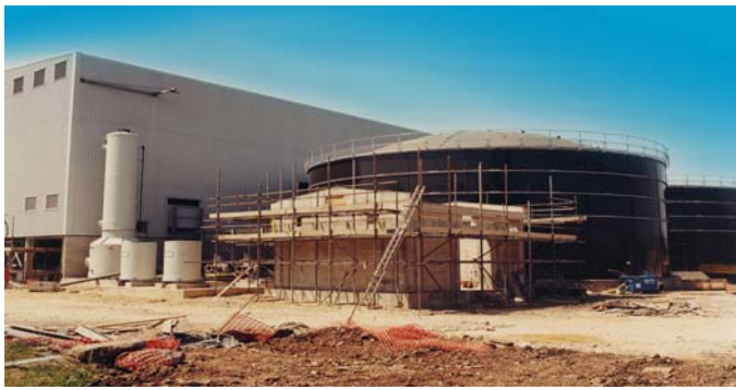
Regenesys Batterie in Little Barford, England 15 MW, 120 MWh
