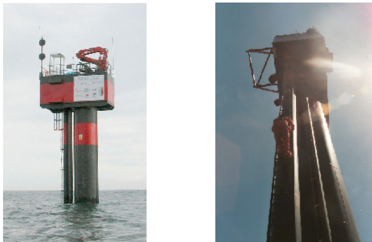
Figure 16: Access, showing the access ladder on separate tube to the pile.
