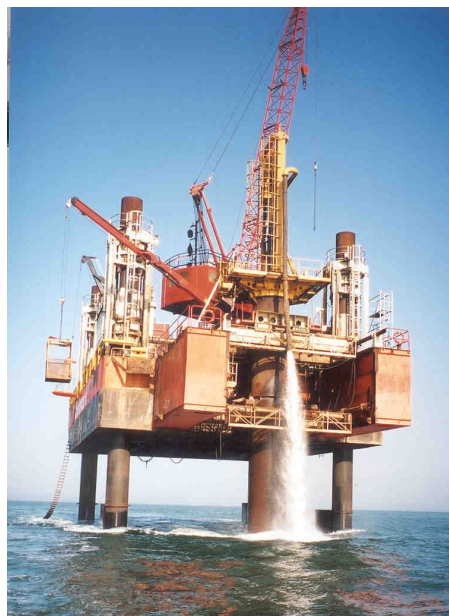
Figure 10: Seacore's Deep Diver jack up barge drilling the socket for the SEAFLOW foundation.
