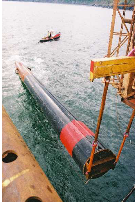
Figure 11: Semi-buoyant lift of pile into the casing.
