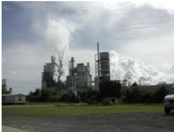
It was developed by Carl Dahl in 1879 and the first kraft mill started in 1890.<sup>1</sup> The invention of the recovery boiler by G.H. Tomlinson in the early 1930s, was a milestone in the advancement of the kraft process.<sup>1</sup> It enabled the recovery and reuse of the inorganic pulping chemicals such that a kraft mill is almost closed-cycle with respect to inorganic chemicals, apart from those used in the bleaching process.
