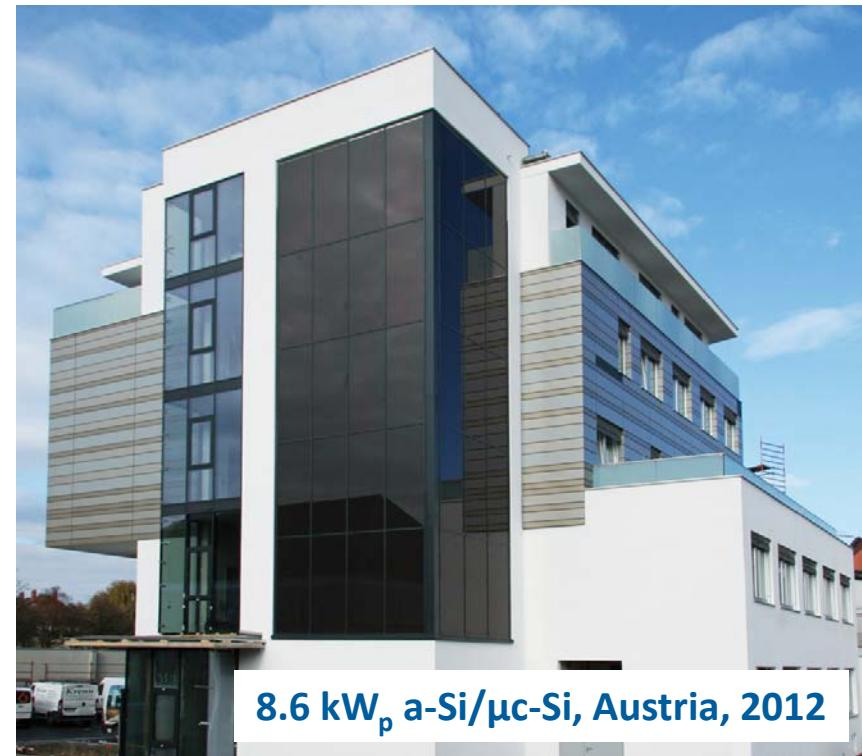
8.6 kW<sub>p</sub> a-Si/μc-Si, Austria, 2012
