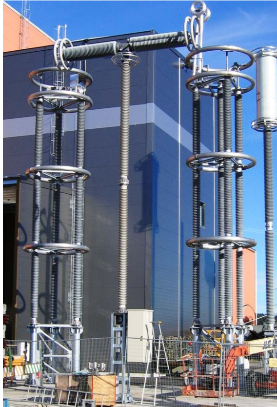
Long-term UHVDC testing after mechanical tests.
