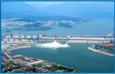
Connecting remote generation
