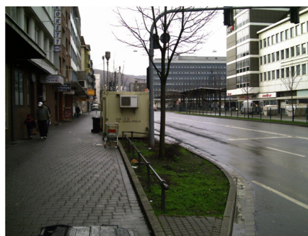
monitoring station in Hagen
