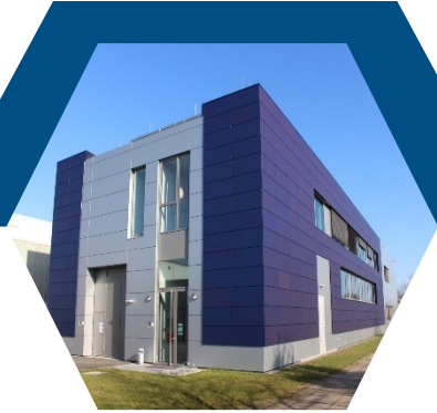
Solar facade at HZB
