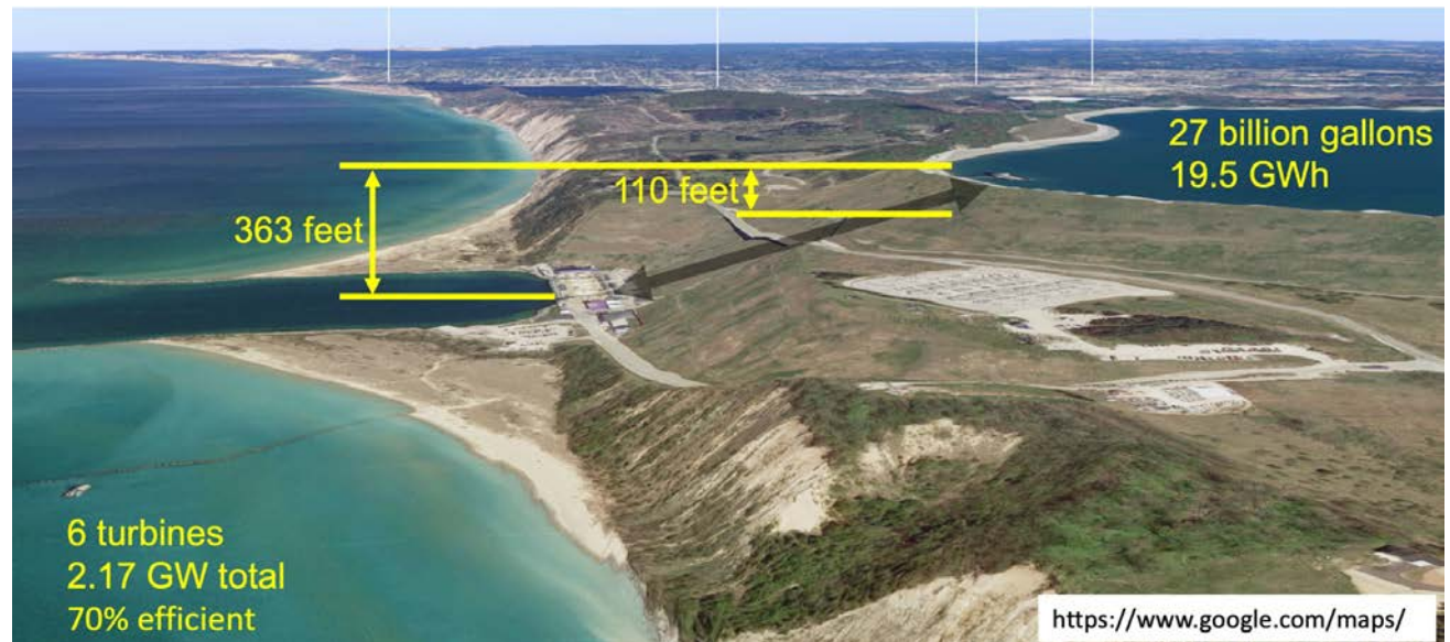
Ludington pump storage plant: Need 200 of these
