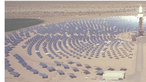
Solarturm in Barstow – Solar Two 10 MW
