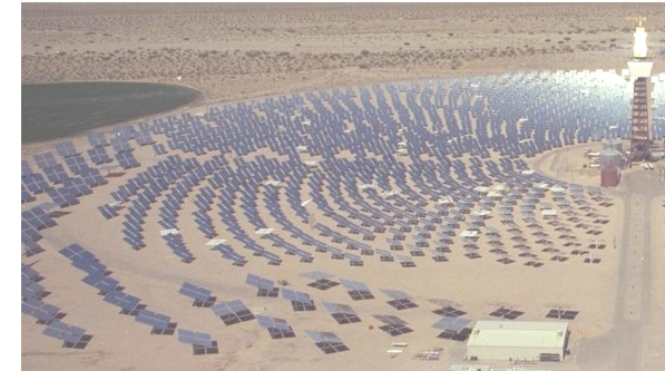
Solarturm in Barstow – Solar Two 10 MW
