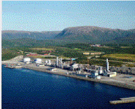
Reformer and gasification plants
