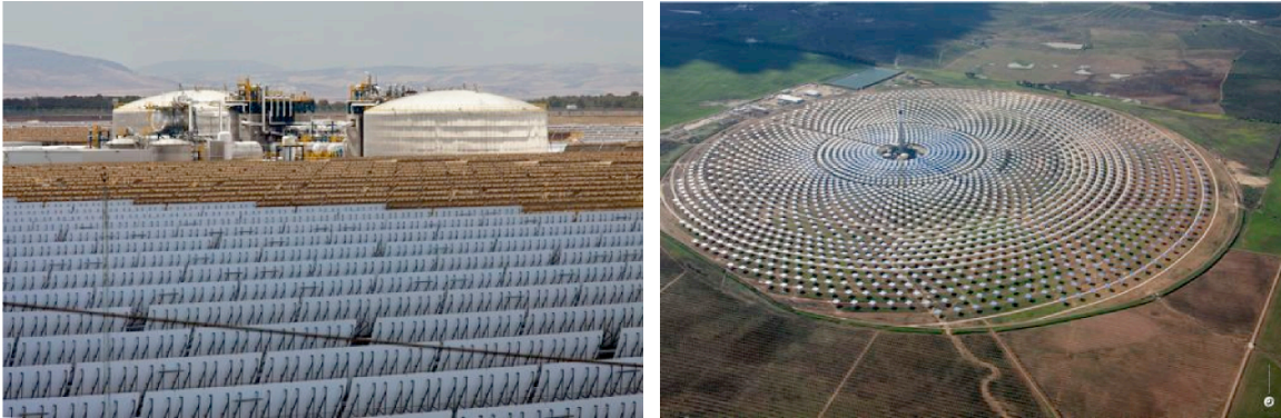
Figure 3: Left: A concentrated solar power station with a field of parabolic troughs (front) and with two large thermal storage tanks (rear). The tanks contain liquid salt that is heated up by the solar field during day. They provide power for electricity production during the night (Photo: Solar Millennium). Right: The 20 MW Gemasol plant in Andalusia/Spain uses molten salt as heat carrier. Storage tanks for hot molten salt permit an electricity generation of up to 15 hours without sun, which allows for an uninterrupted operation day and night (Photo: Torresol Energy).
