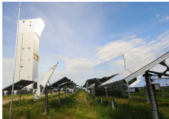
Solar thermal power plants
