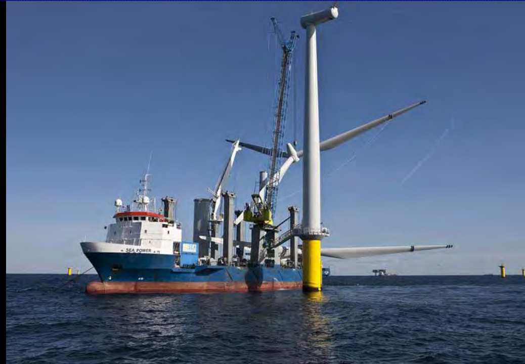
2.3 MW turbine: 93 meter diameter blades, 115 meters high.
