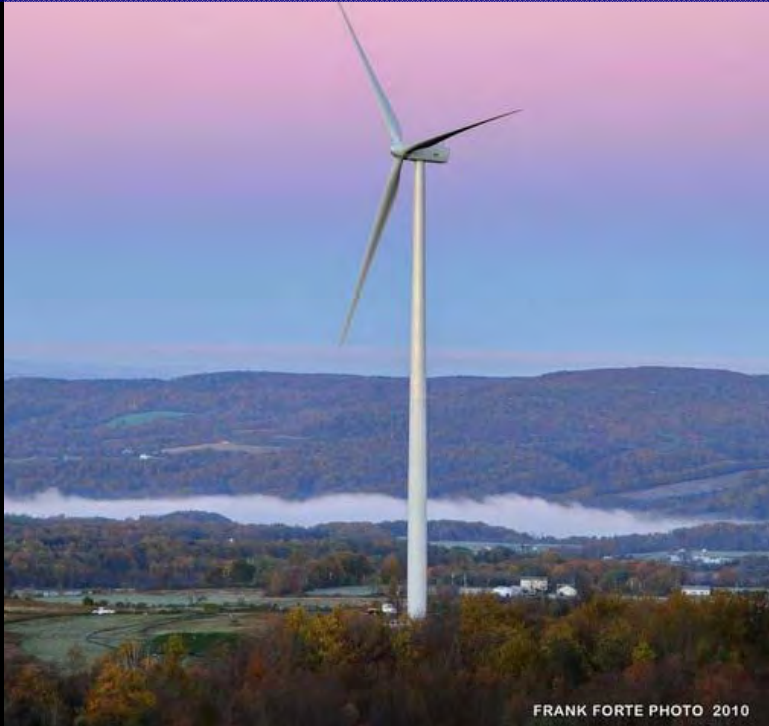
100 meter wind tower
