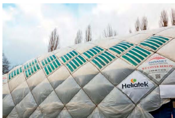
Fig. 8: Concept for an energy self-sufficient air dome. Picture source: [1]
