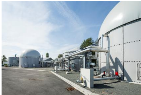
Biogas pilot plant (75 kW eI )
