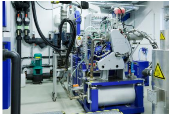
Engine test bed
