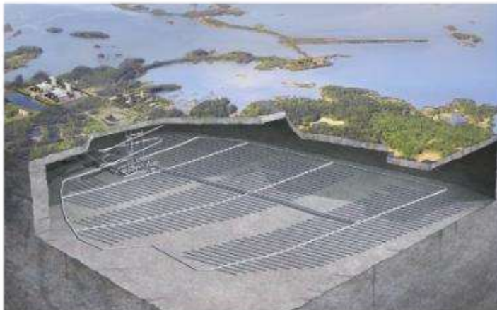
An artist's impression of the planned repository concept, with its 66-kilometre network of underground tunnels (Image: SKB)
