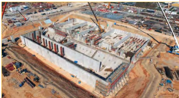
Fig. 14: ITER power will be partly evacuated by cooling towers (procured by India). Here: construction of the building for the cooling water system with "hot" and "cold" basins. (Source: ITER)
