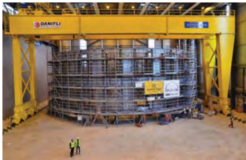
Fig. 13: On-site assembly and welding of the cryostat lower cylinder from elements manufactured in India. (Source: ITER)
