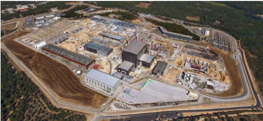
Fig. 1: Aerial view of the ITER site at St.-Paul-lez-Durance. In the centre of the photograph is the assembly building (dark) and behind it the tokamak complex under construction. In the foreground, left, the 250 m long building for the winding of the poloidal field coils. (Photo: ITER)
