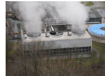
Power stations: hydropower and cooling water
