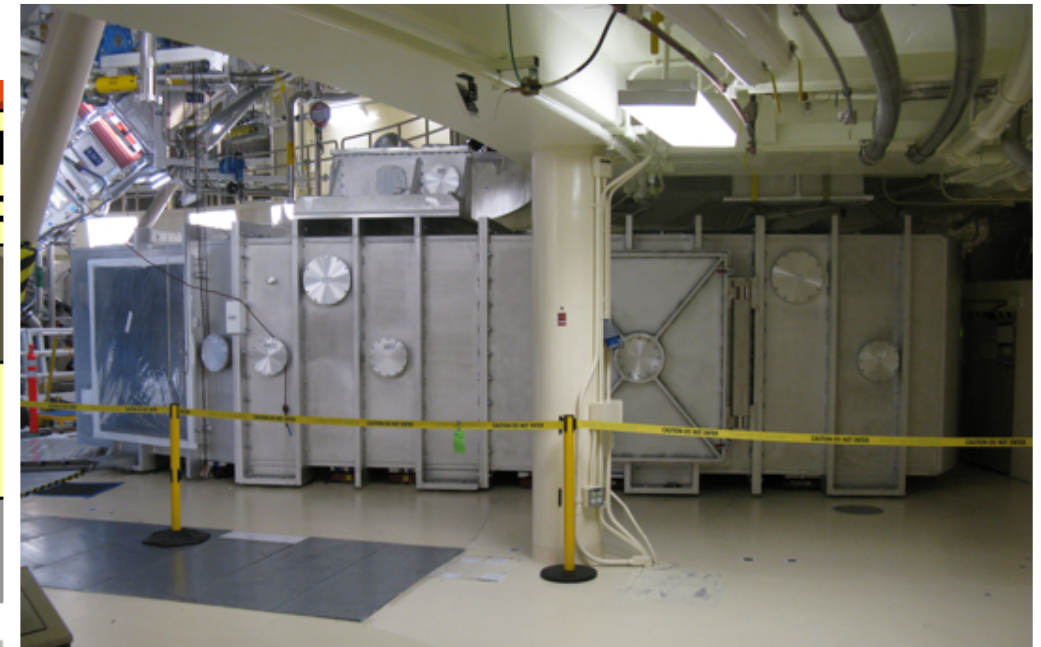
Compressor installed in target area
