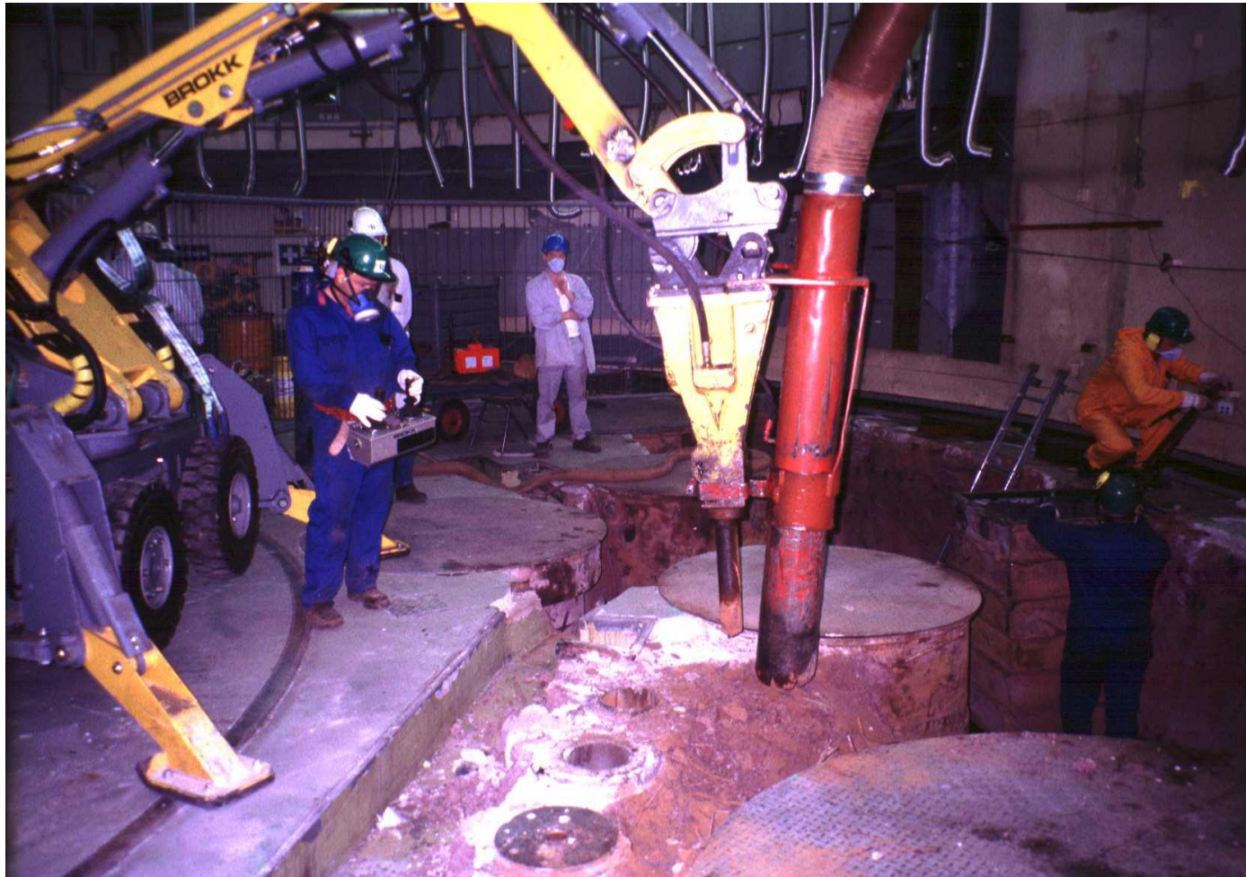
Dismantling and extraction of heavy concrete with chisel and suction pipe
