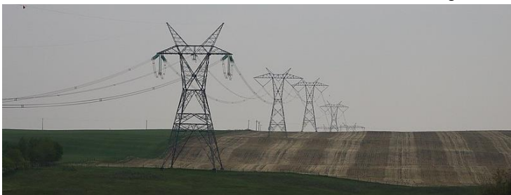
HVDC transmission line by TagsSanPedroAko, licensed CC0, via wikimedia.org .
